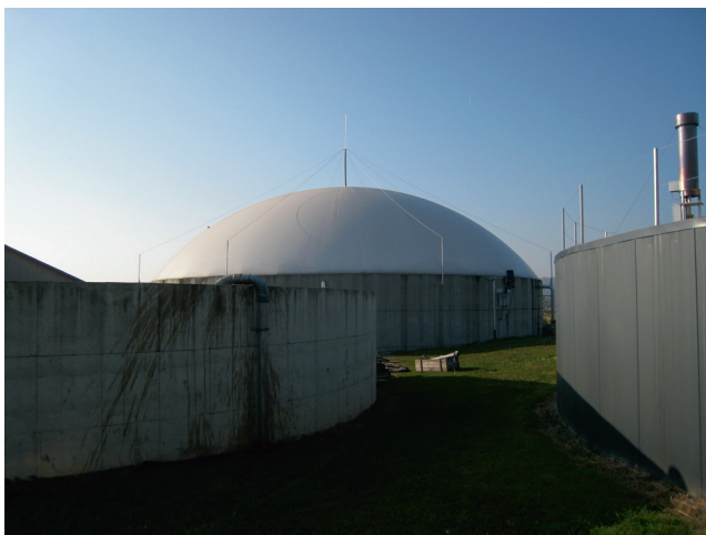
Figure 45: Biogas plant/fermentation tank with foil gas storage
