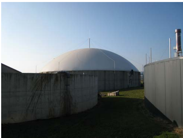
Figure 45: Biogas plant/fermentation tank with foil gas storage
