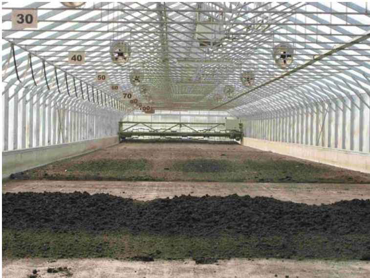
Figure 72: Solar sewage sludge drying plant, waste water association Leibnitzerfeld Süd
