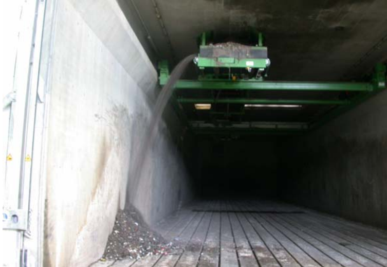
Figure 22: Intensive rotting tunnel, MBT Frohnleiten
