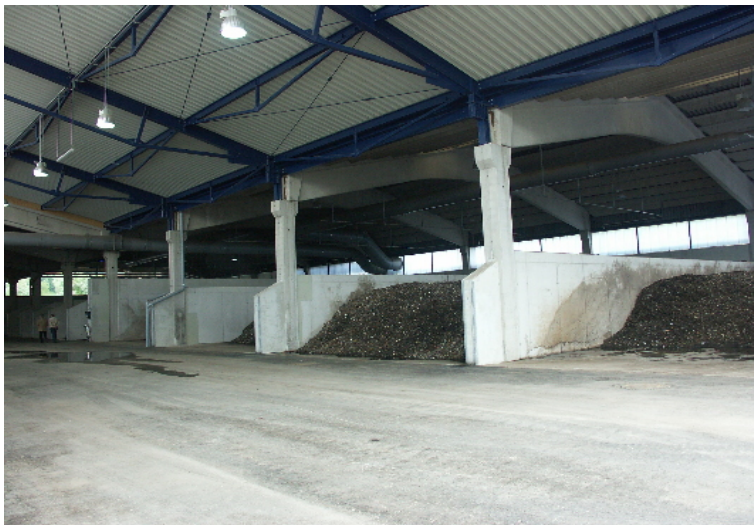
Figure 23: Post-rotting, MBT Liezen
