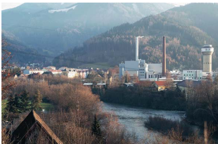
Figure 26: Thermal residual waste recovery of ENAGES in Niklasdorf
